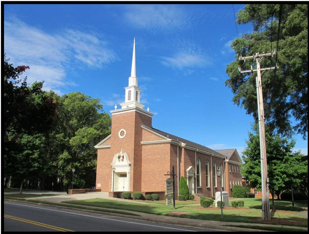
Figure 2.2-17: View of the Huntersville First Baptist Church of 1962, Looking Southwest.
