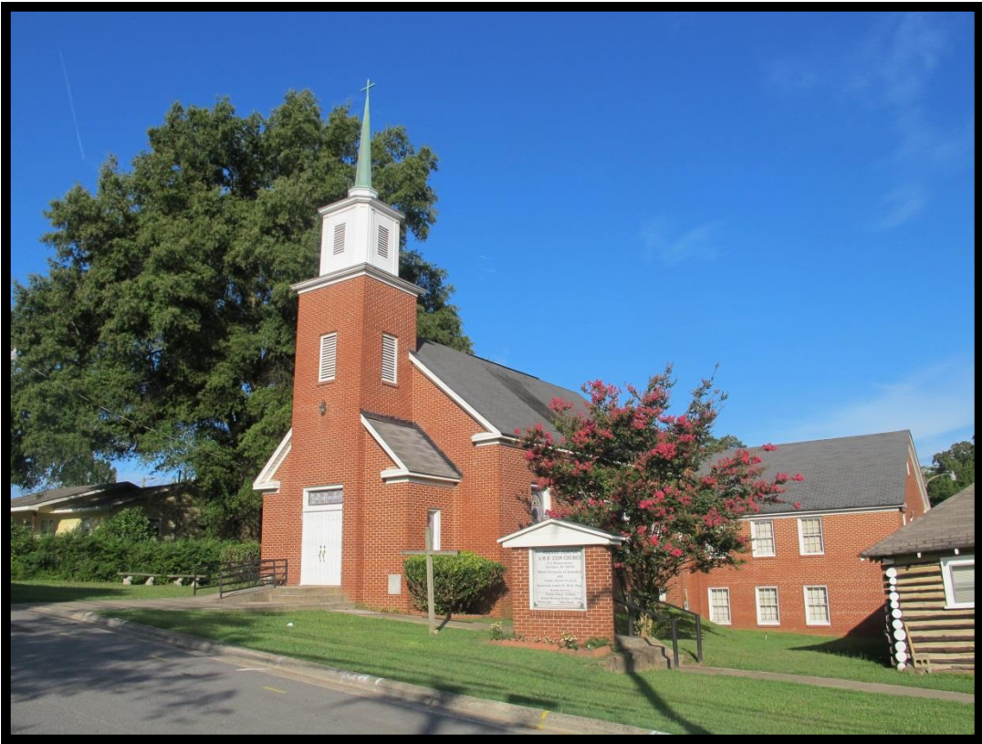
Figure 2.2-19: Reeves Temple African Methodist Episcopal Zion Church in Davidson, ca. 1965, Looking Southwest.
