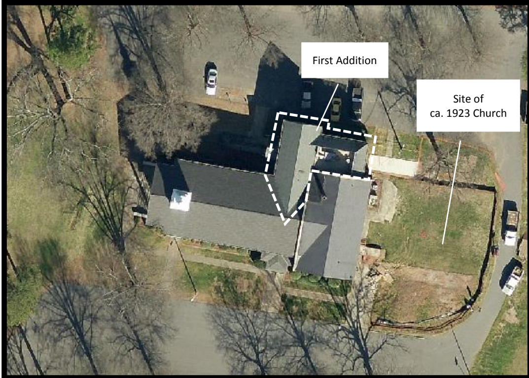
Figure 2.2-15: Detail of 2012 Aerial Showing the Huntersville Associate Reformed Presbyterian Church (MK1342) (Polaris 3G 2016).
