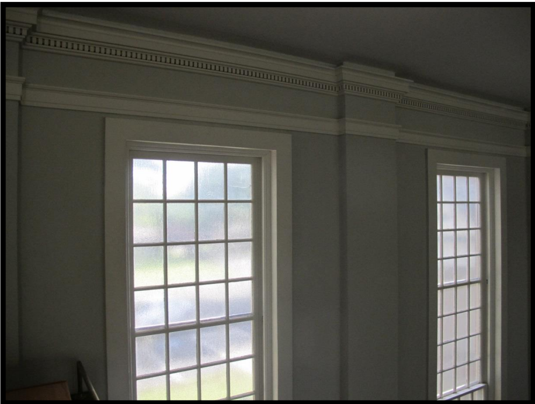
Figure 2.2-8: Church Interior (MK1342), Detail of Entablature on North Wall.
