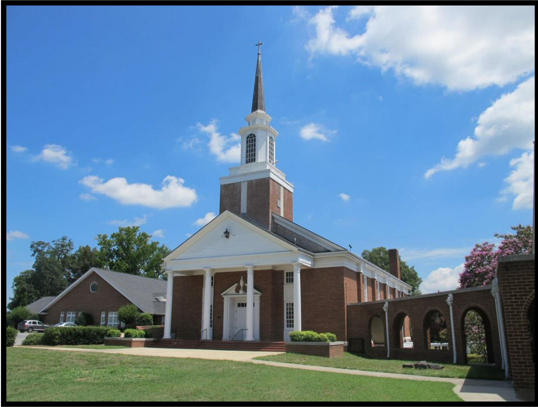
Figure 2.2-21: Back Creek Associate Reformed Presbyterian Church in Charlotte of 1970, Looking Northeast.
